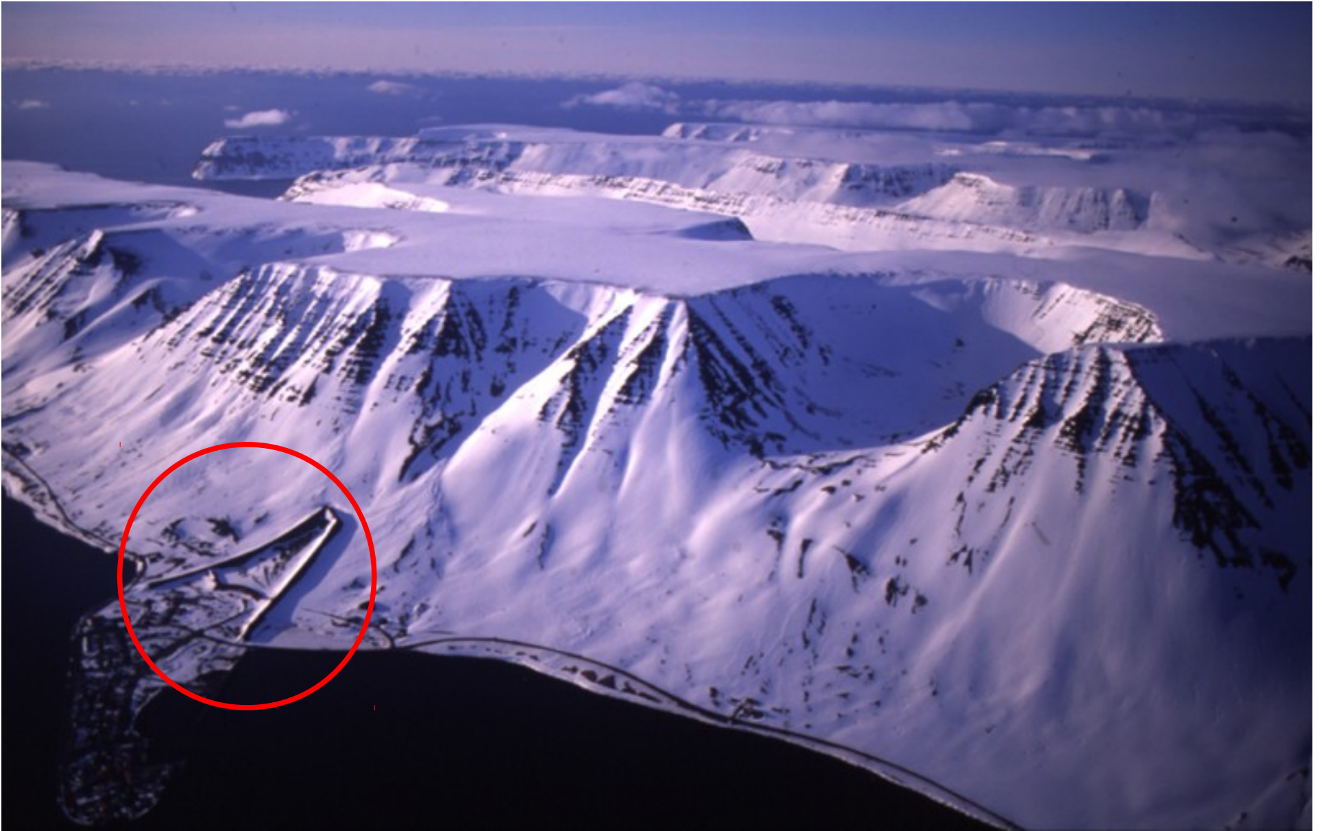
Deflection dam system protecting Flateyri, NW Iceland
