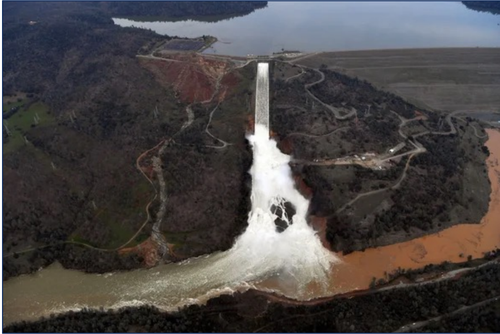
Oroville Dam spillway overflowing in February 2017 following an atmospheric river event in California.
