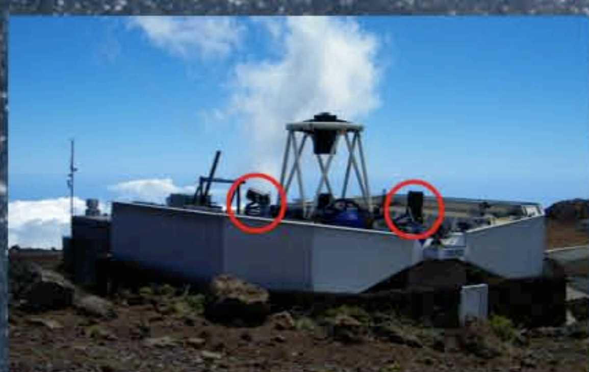
Figure 1: The 2m FTN at Mt. Haleakala, Maui, Hawaii. Two 0.4m telescopes, encircled in red, are located within the clamshell dome. Those are the network's first 0.4m telescopes that have been deployed, currently being commissioned.
